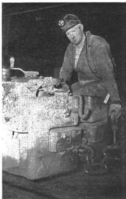
George Schmitt of Iroquois Shaft with car coupling showing the safety handle he devised.
