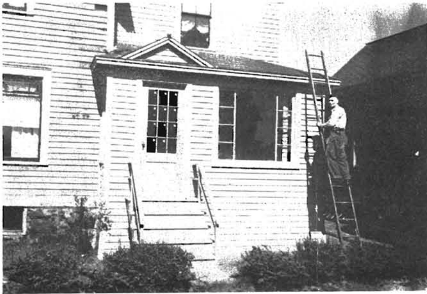
Having completed building an enclosed porch, Joe Notario of the Foundry does a paint job on his house.
