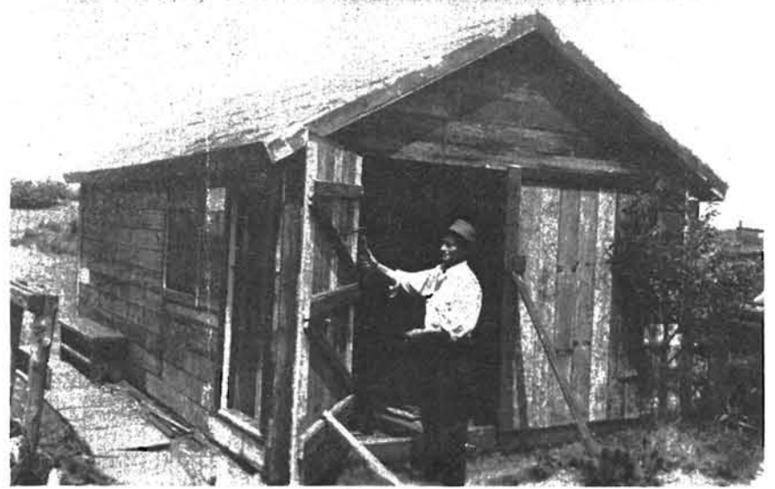
George Geshel of No. 4 Kearsarge building a garage.
