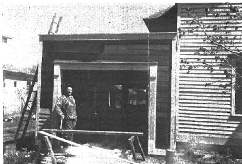
Herman Anderson of the Roundhouse building a garage.
