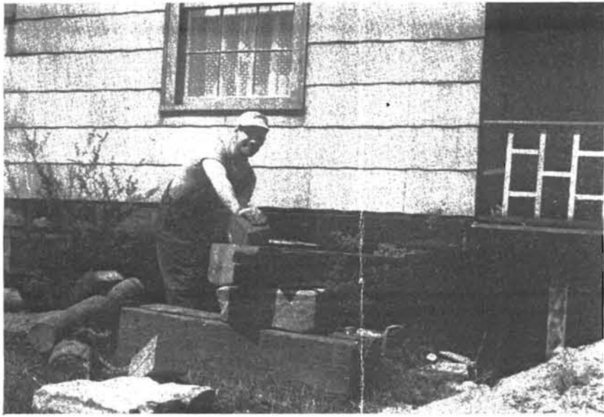
Oliver Michaud of the Ahmeek Mill excavates for a foundation and basement under his house.
